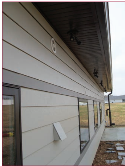
Photo 4 (left): Exterior view of the fresh air supply vent (lower) and exhaust air vent (upper) on the north side of the house. Note the specially designed downspout at the end of the house for rainwater harvesting from Equinox's steel roof. Photo 5 (right): Remote control switch used for zero wall penetration, exterior lighting circuits.
