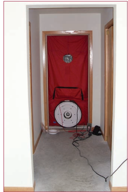
Photo 1: Blower door in garage door.
