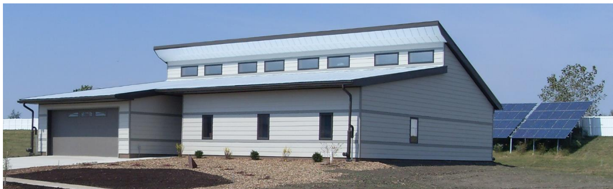
Figure 1 Photograph of Equinox House in 2011 near the spring Equinox. Note the clerestory shading of the upper “Equinox overhang”. During winter, the white, uplifted overhang and the 2/12 pitch, white roof below concentrate solar radiation on the clerestory. The overhang excludes direct solar radiation (85% of clear sky solar energy) from spring equinox to fall equinox.
