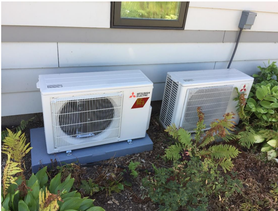
Figure 3 Equinox House has two ductless minisplit heat pump units. The outside units with compressor and outdoor heat exchanger are identical for ducted and ductless heat pumps. Read our “Minisplit Mania” news article and related report to learn why two heat pumps are more efficient than one!
