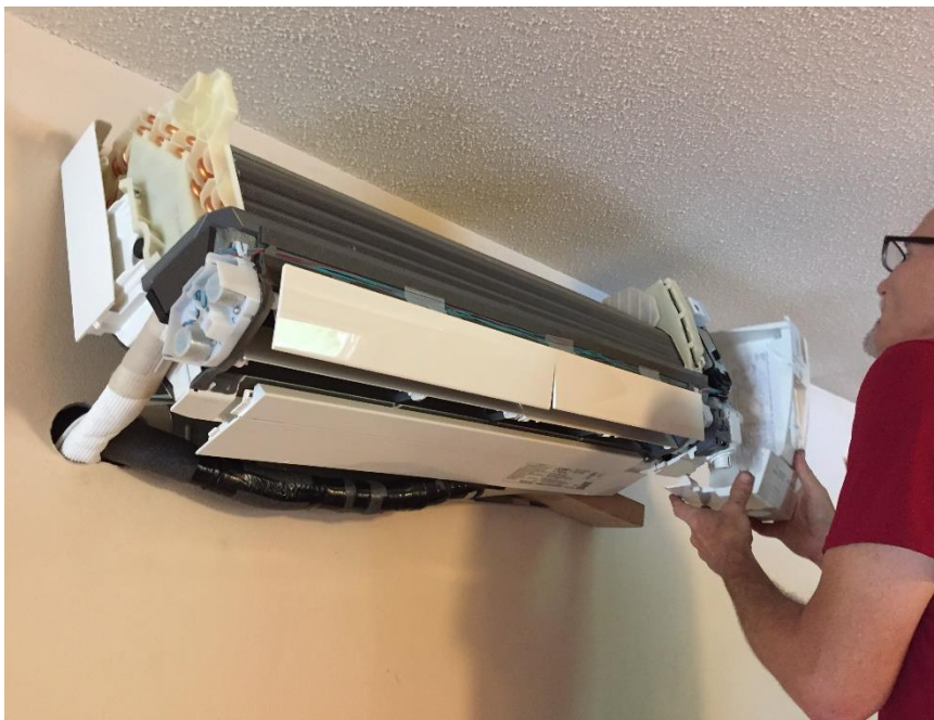
Figure 1 Indoor heat exchanger for a “ductless” minisplit heat pump. During summer operation as an air conditioner, the heat exchanger is cold and condenses water vapor. The white insulation clad tube on the left is the condensate drain tubing.
