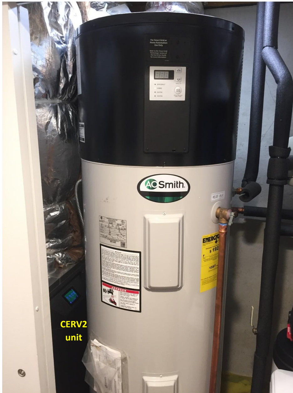
Figure 15 HPWH installed in a small mechanical closet adjacent to a CERV2 (left) smart ventilation unit. The CERV2 allows the HPWH to be placed in a small, enclosed space.
