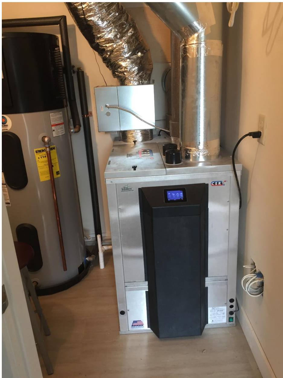
Figure 25 A second generation CERV2 in a small mechanical room shared with a HPWH in a high performance Vermod home . The HPWH and CERV2 share a condensate drain (white plastic pipe between the units).
