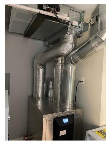
If the system to be controlled by the CERV-IR-T is a ducted heat pump, and the inlet of the heat pump is directly connected to the outlet of the CERV, an Outlet Temperature Probe is required to ensure synchronized defrosting between the two units. This section may be ignored if this scenario is not applicable.
