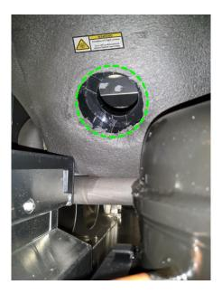
The UV lamp socket should now pull out of its plastic base. Take note of the orange latch on the mount, as well as the notches in the plastic base.
