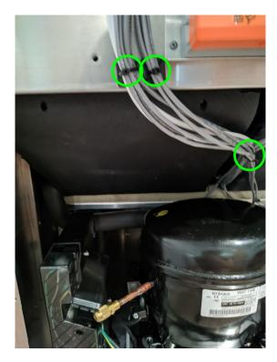
If there is not enough slack in the CERV2's wire harnesses, the zip-ties highlighted above may be clipped, allowing them to be moved further out of the way of the access panel when removed. If the zip-ties are removed, use the kit's included zip-ties to secure the harnesses again once installation is completed.
