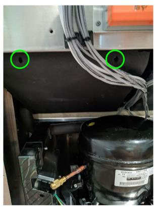
Using the 1/4" Driver, locate the two hex-head screws at the top of the access panel, and unscrew.
