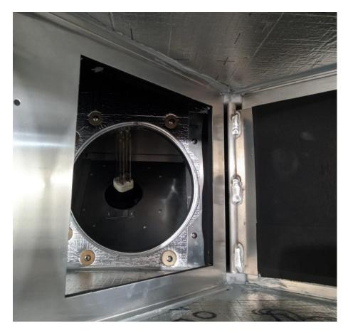
Looking down (from the front of the CERV), the newly installed UV lamp should be visible. If the damper paddle is covering the opening DO NOT FORCE IT BY HAND! To move the damper paddle, turn on power to the CERV, and make sure CERV operation mode is set to off. Wait for damper to move into position, then turn power back off.
