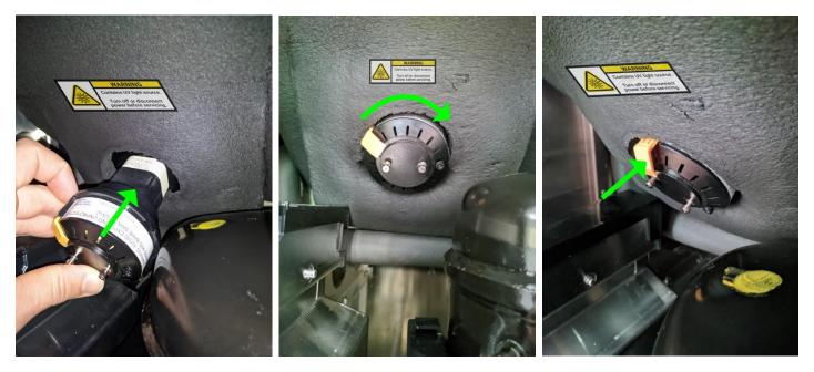
Carefully insert the UV lamp/socket into the plastic base (aligning the notches), then rotate approximately 30 degrees clockwise and press in the orange plastic clip. The mount should now be securely held in place.
