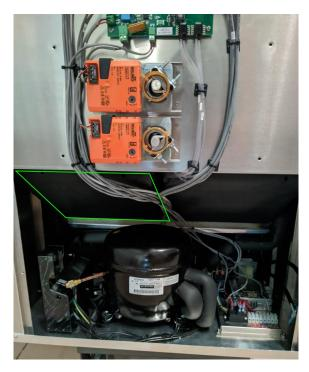
With the front enclosure and lower access panel removed, locate the duct access panel on the left side outlined in green above. This is the Supply duct for the home, and will receive a new duct access panel with the UV lamp mount.
